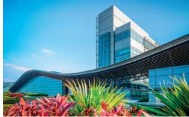
The surplus electricity exported to the public grid by T•PARK, which has a treatment capacity of 2 000 tonnes of sludge per day, is sufficient for use by about 4 000 households annually.
