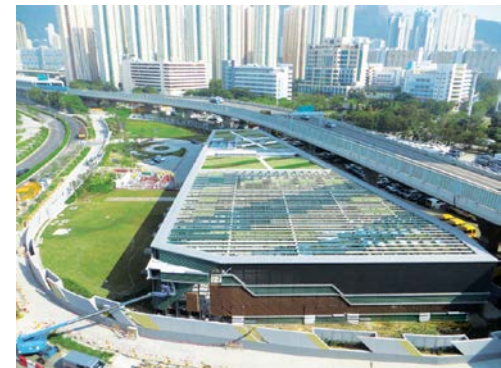
District Cooling System at Kai Tak Development
